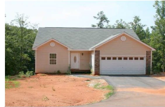
1619 Butler's Bridge Road McDonough, GA 30252 $93,000.00 Contact Kenneth Howell Bank will finish
